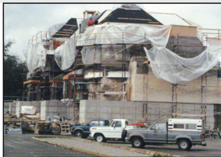
1992 Roofing the Museum in the Northwest rain.
